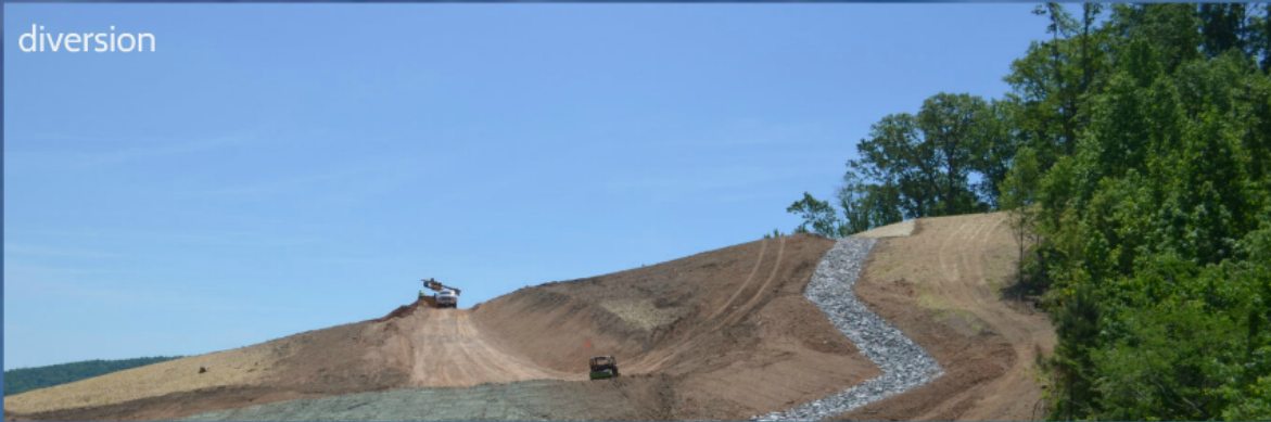
early installation of cross-drain
