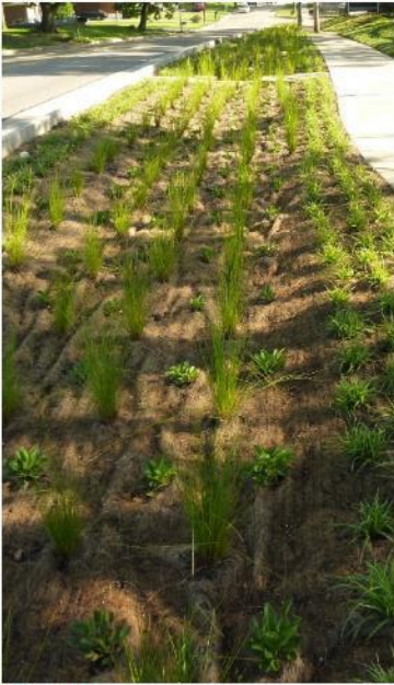
FIGURE 3-7 ▲ NEWLY-INSTALLED BIOSWALE WITH RIGHT-OF-WAY
