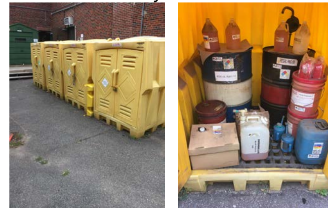
Covered secondary containment
