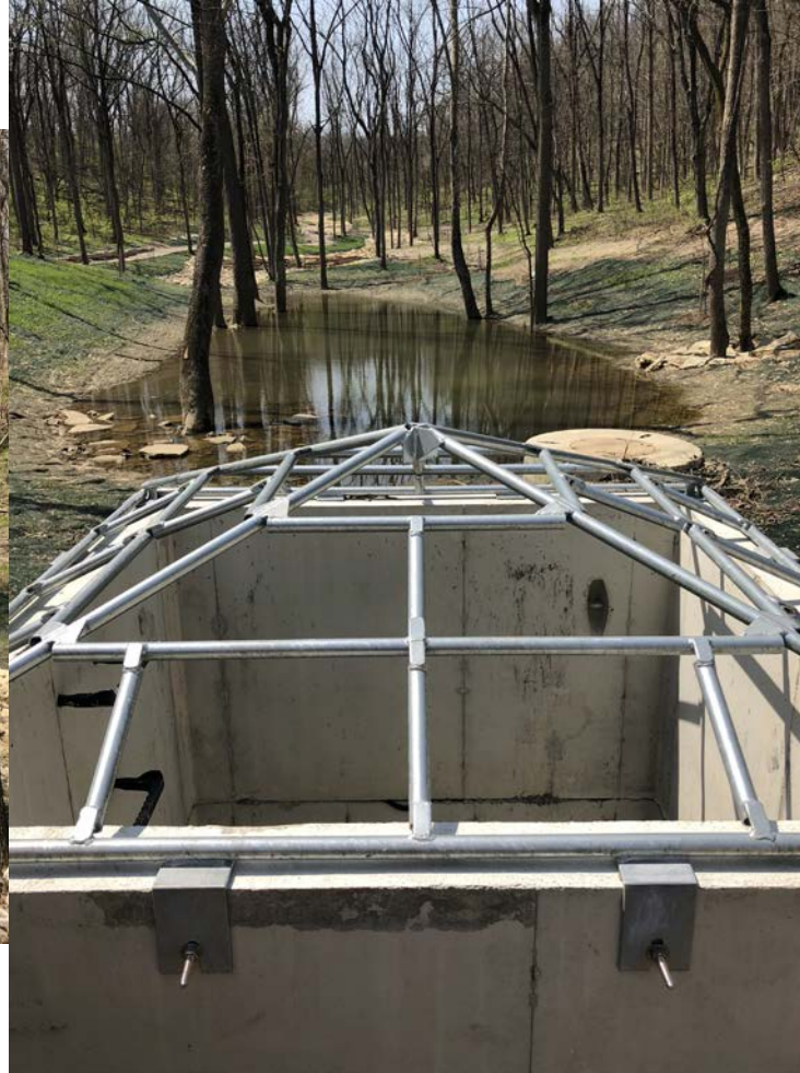
Detention Outlet Control Structure
