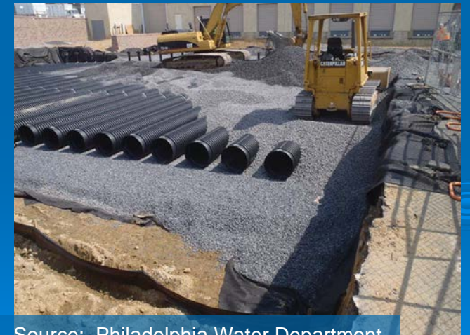
Underground Infiltration System
