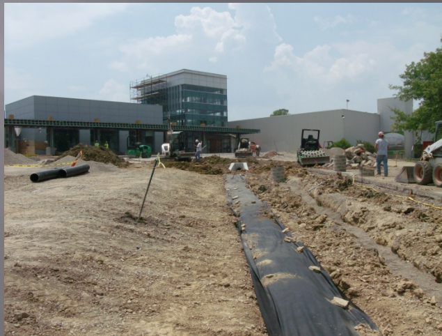
Underdrain Installation
