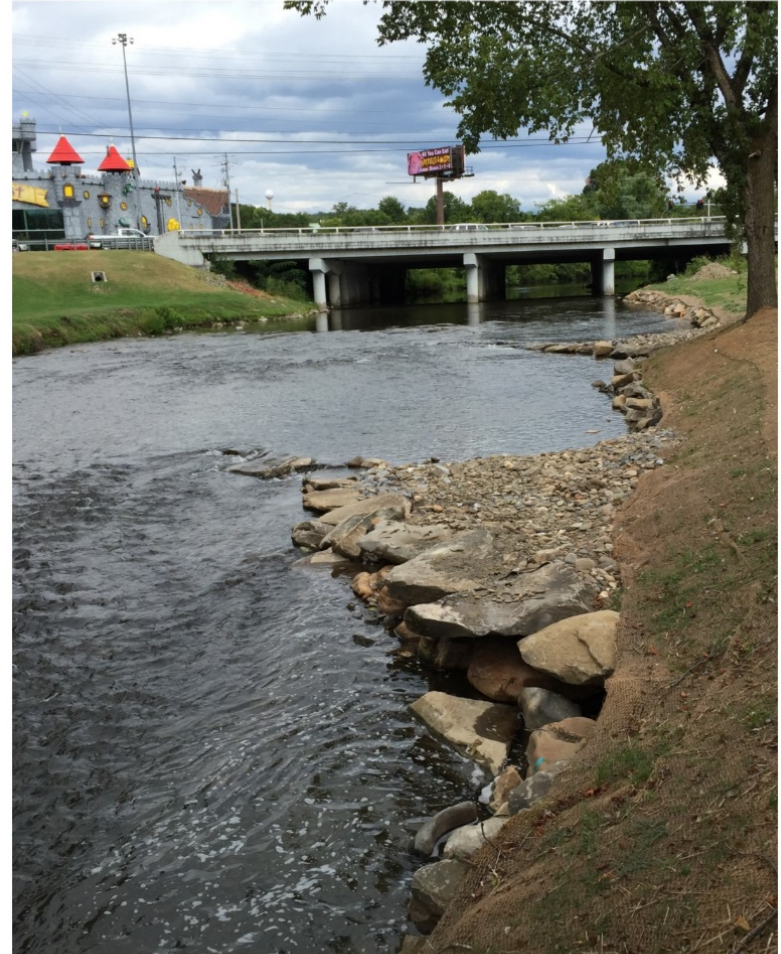
Photo 1, After: Completed Bank Work and Installed Rock Vanes Following Construction
