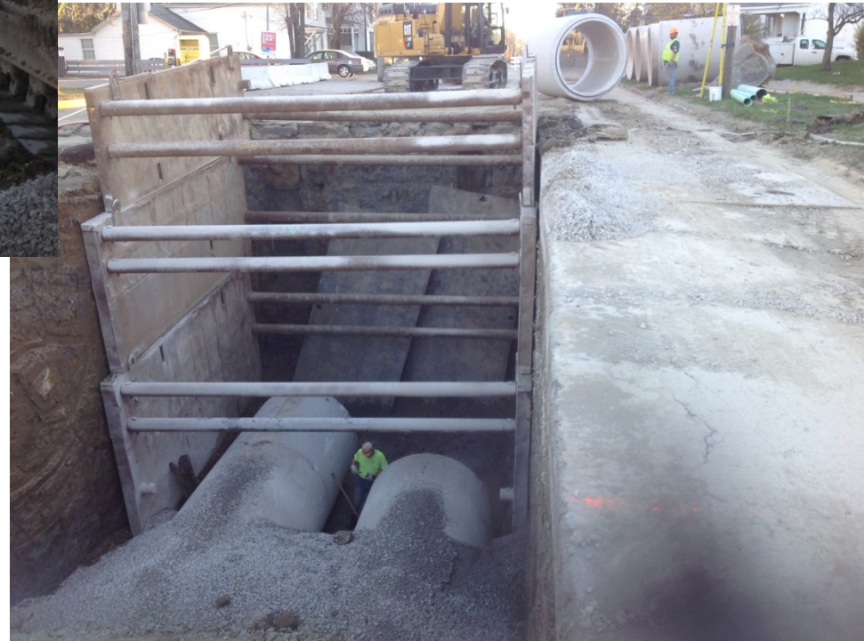
In-Line Storage at Downstream End
