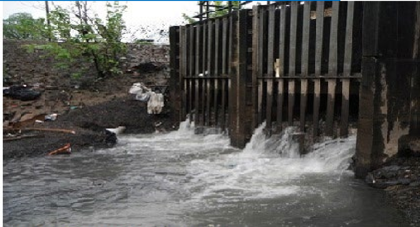
Combined Sewer Overflow; Photo credit: EPA
